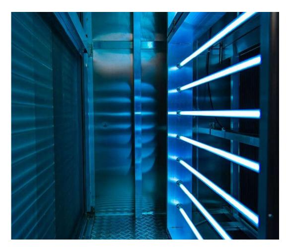
UVGI lamps exploit the advanced technology of UV-C rays, which are able to eliminate pathogenic elements such as viruses and bacteria.
